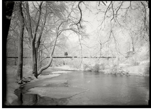
Cowles Lodge Bridge, 1929
