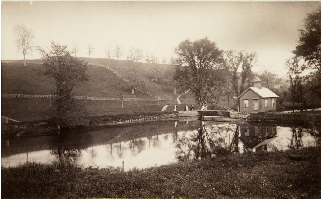
Prospect Hill and Pump House from Northwest, 1884-86
