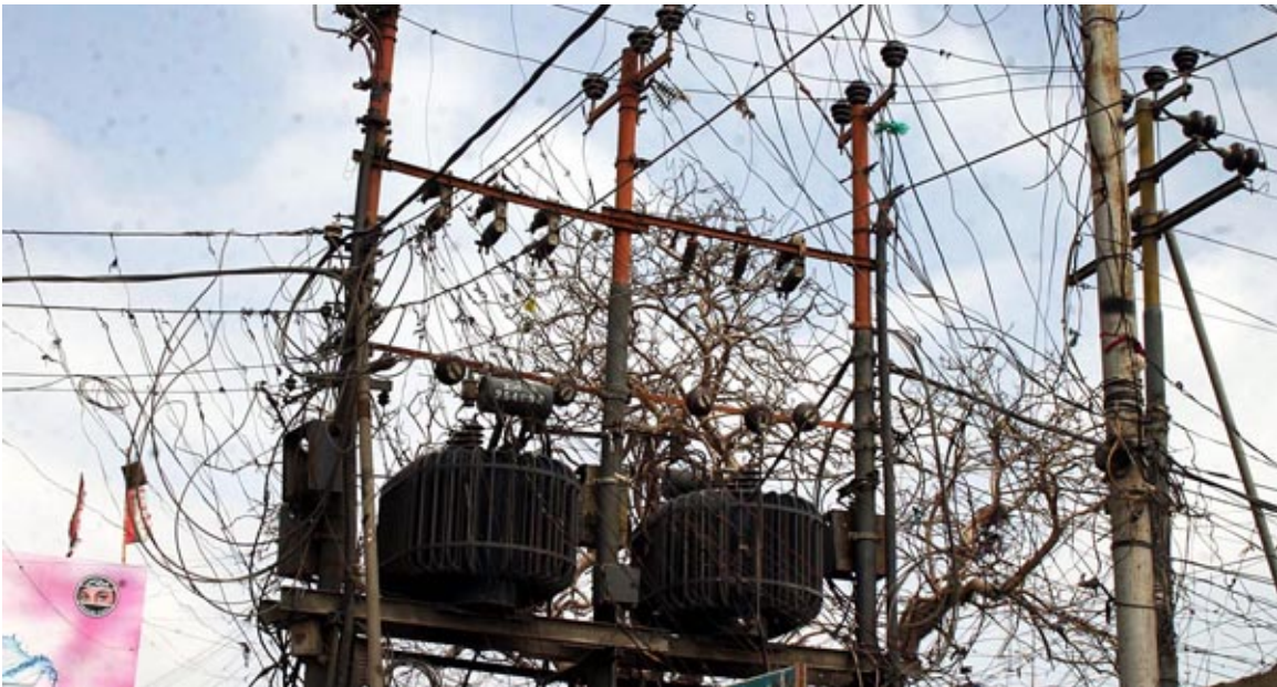
Figure 1-1: (a) The commercial center of Karachi. The city consumes 25 million kWh at peak consumption which levels out to an average of 60 million kWh over the course of the day. (b) Transformers often burn out under the load of all the illegal connections that find their way onto the pylons.
