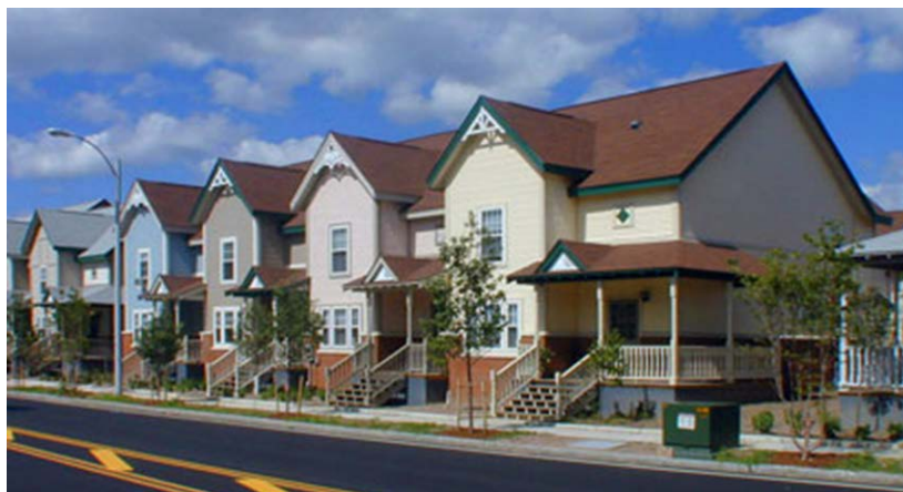
Figure 7. HOPE VI Rebuild of Jackson Parkway
