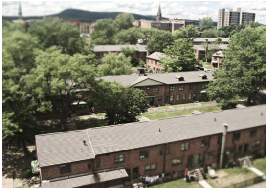
Figure 5. Aerial View of Lyman Terrace
