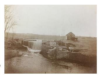
summer, modifications were made to the dam to prevent future flooding, namely a 10 foot widening of the dam opening, to allow more efficient water flow out of the lake during flood events (3). The Dams are now subject to inspection every other year, and repaired as needed. The water level in Upper Lake can be controlled manually using a sluice gate. This mechanism is to be updated by the end of June, 2018.
