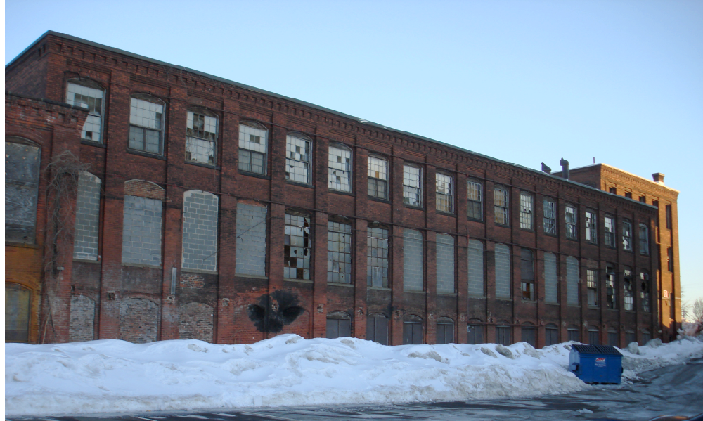
First group of buildings, more modern in style
