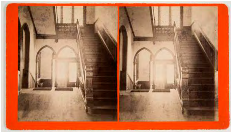
Stairwell, first floor
