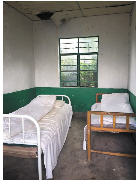
Dilapidated treatment room
