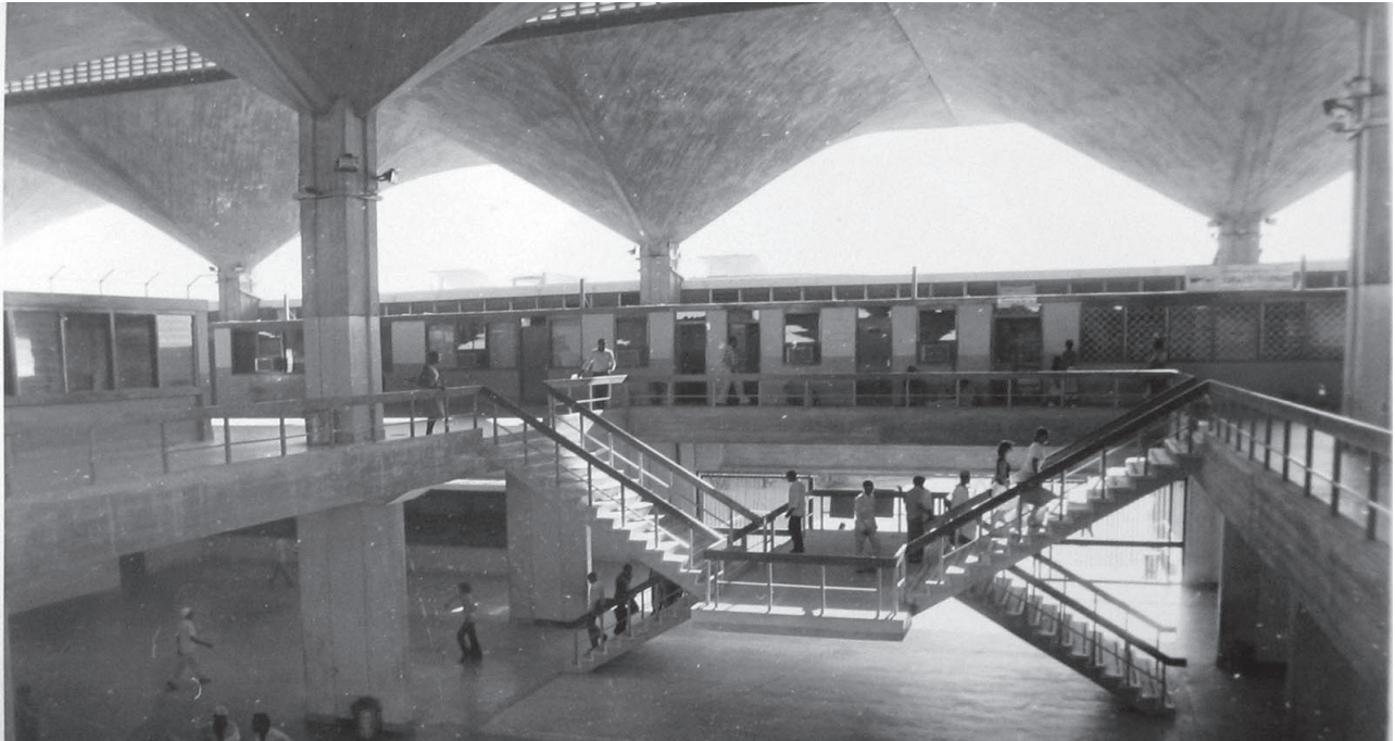
Photo of the interior of the new market building in Kariakoo on the day of its inauguration, 1975. Photo from the private archive of Beda Amuli.
