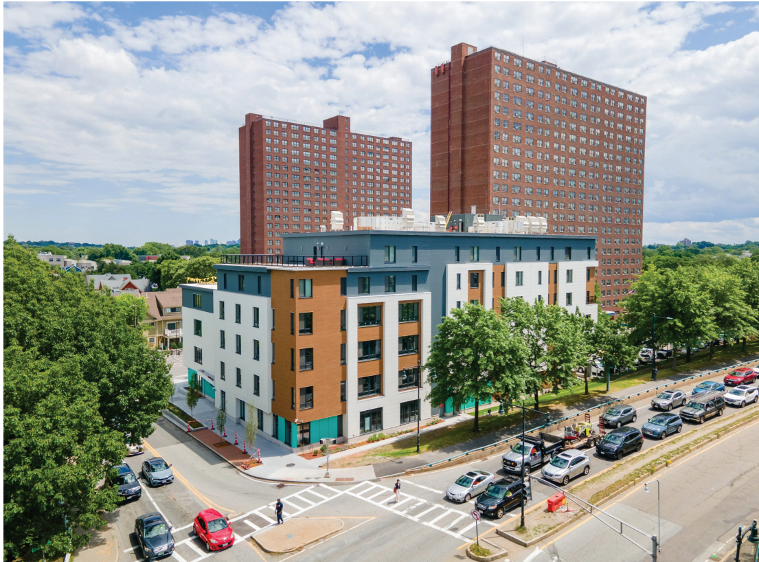
Part one of the Rindge Commons development – Rindge Commons North, completed summer of 2024. Image from Dellbrooks JKS Developers.
