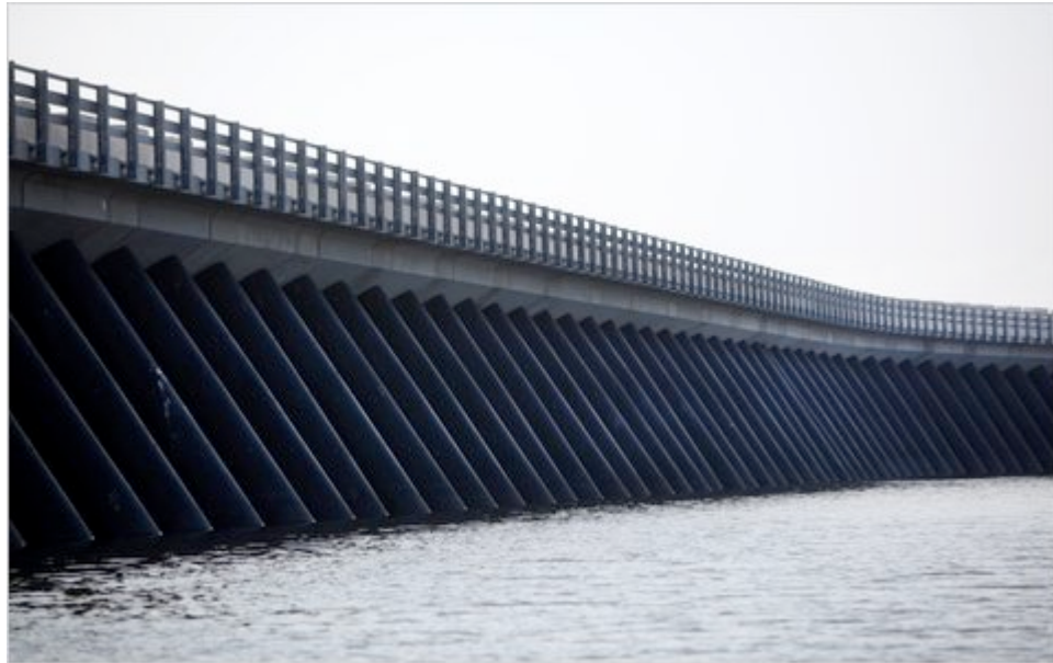
Figure 1: New Orleans Levee System 2010
